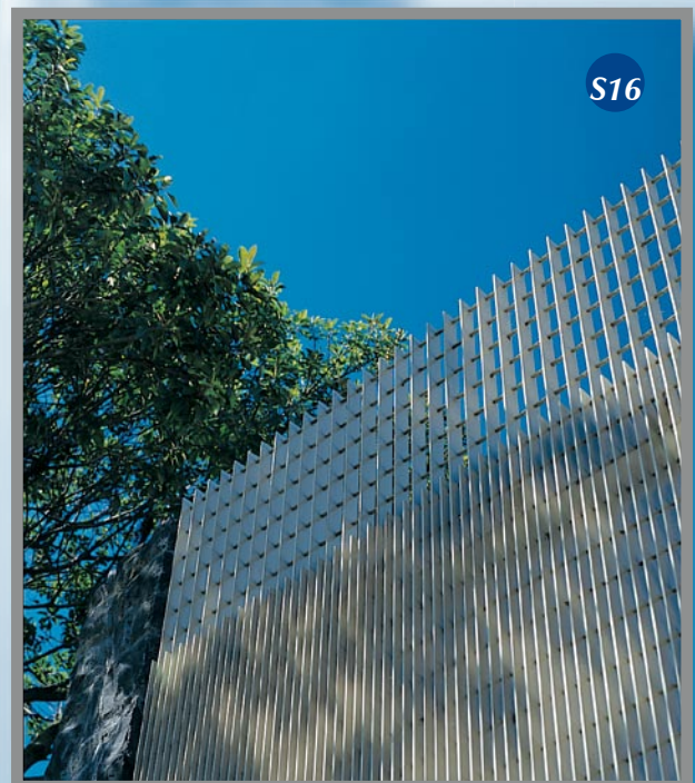
Homebush Substation, Homebush, NSW, HA505 and HC505 combination grating patterns create a picket fence and gate attached to structural framing and electronic door-locking mechanism.
