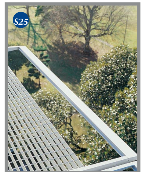
Rushcutters Bay Hotel, Sydney, NSW, HC753 grating, DAN019 outrigger and DAN023 nosing.
