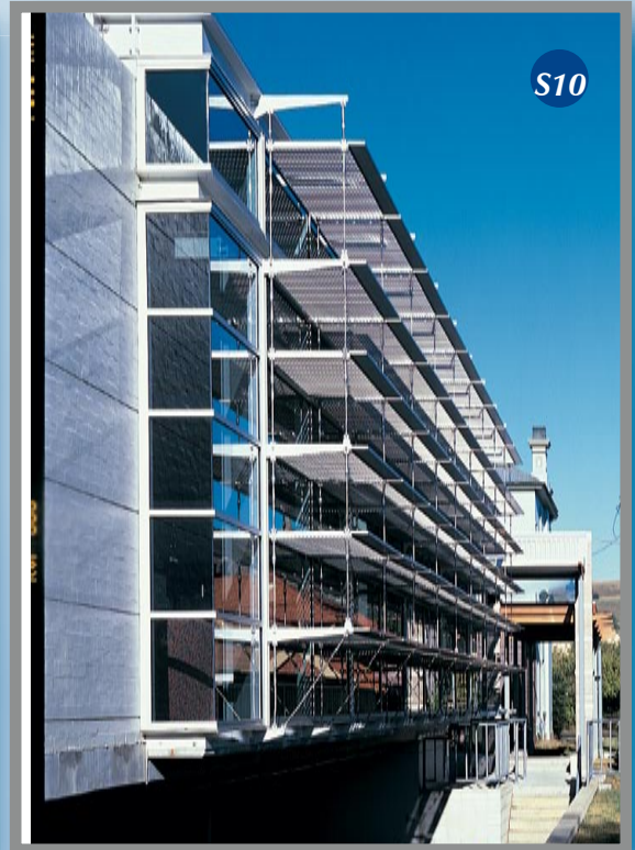
Bowral Library, Bowral, NSW, HA503 grating with RHS nosing, suspended and tensioned with stainless rod hangers and attached to structural window framing.
