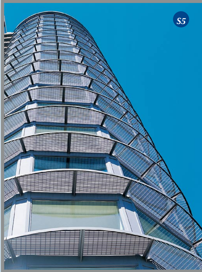
The Pinnacle, North Sydney, NSW, HA503 grating and aluminium "T" section support framing. Access to the platforms utilises abseiling technique.
