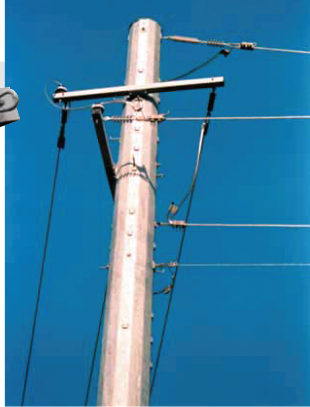
8' braceless 10,000# Dead End assembly, 373' of 795 AAC
