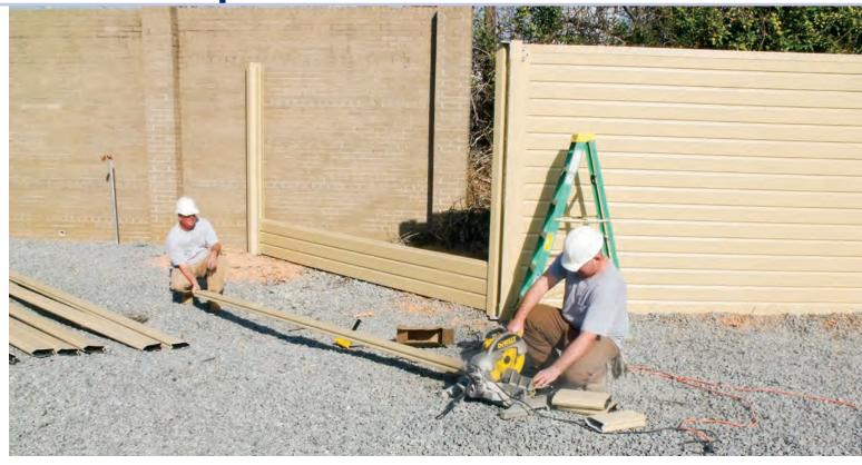
Carsonite sound barrier planks are adjustable and can be easily cut in the field.
