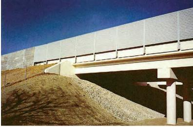
At only 5 to 7 pounds per square foot, AcoustaShield does not add unnecessary weight to bridge structures.
