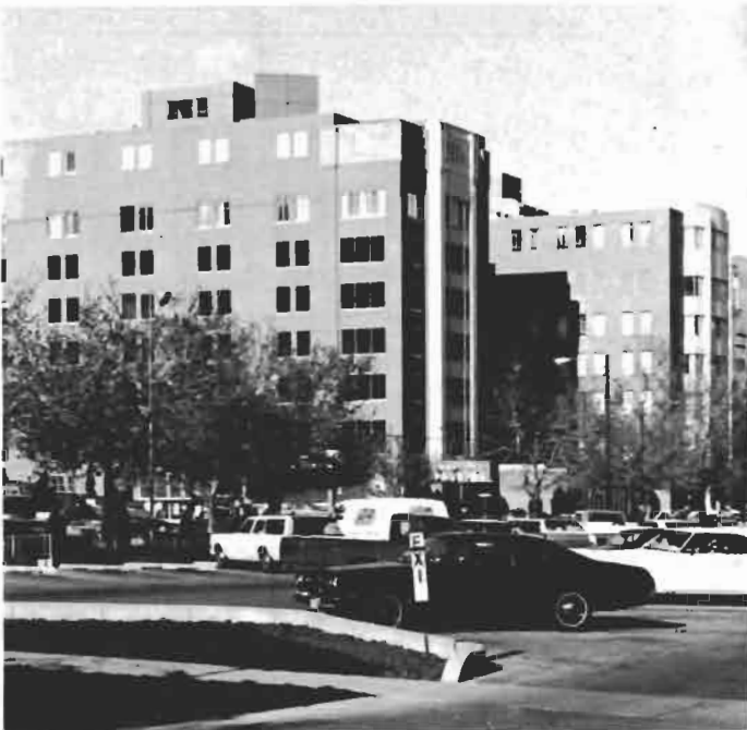
Building mounted passive repeater
